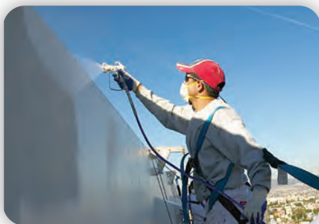
Machine application using Graco airless sprayer
